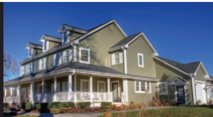
In seven days, a 3,200 square-foot home in Dundee, Wisc., was built for a local family in need, with $25,000 in electrical materials provided by Hein and other distributors.
